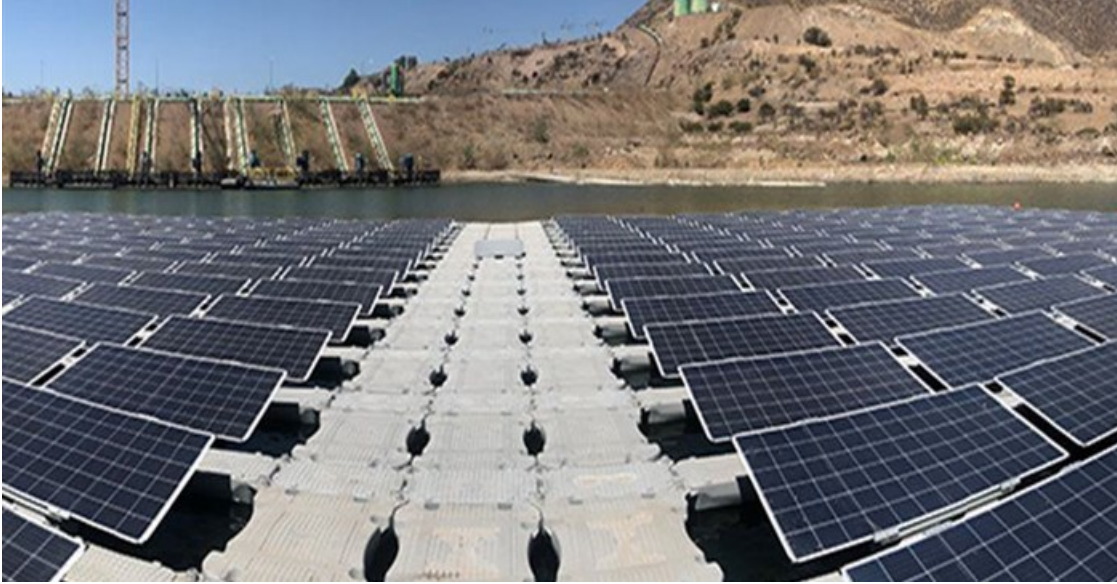
Anglo American built a photovoltaic plant over a tailings dam at its Los Bronces copper mine in Chile
